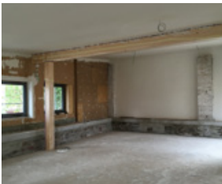
UdiSUN® in the ceiling coated with filler
