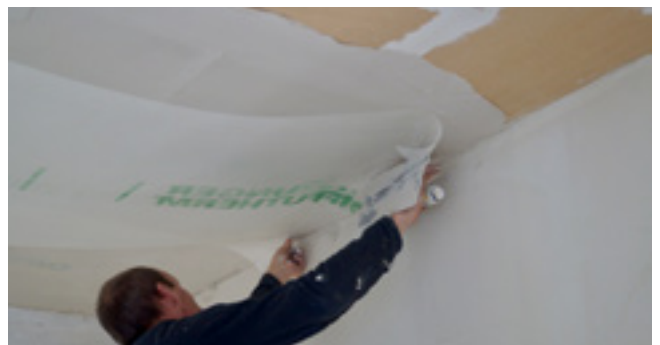
Install the reinforcement mesh in the same way
