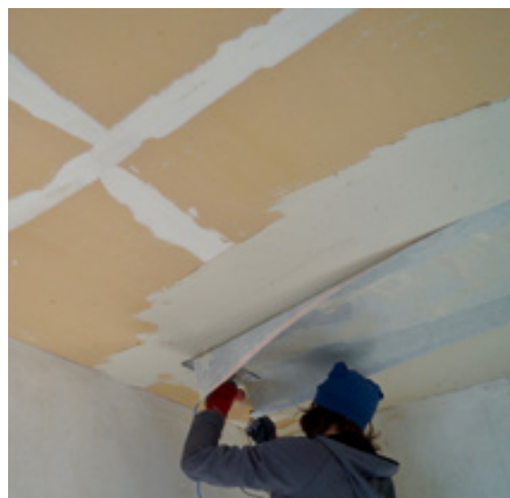
Apply the UdiSUN® heating sheet
