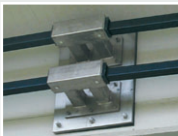
▲ Duct fixings for bridge tensioning constructions
