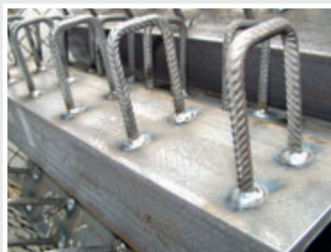
▲ Mounting bracket with reinforcing bar brackets
