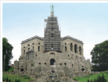
▲ Herkules, Bergpark Kassel-Wilhelmshöhe: Supports (foundation ring), reinforcements and figure supporting structures
