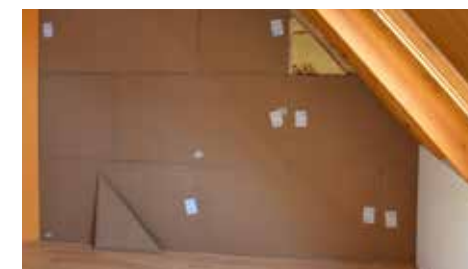
Wall insulation PhoneStar ST
