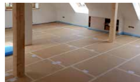
Loft conversion PhoneStar installation in one layer
