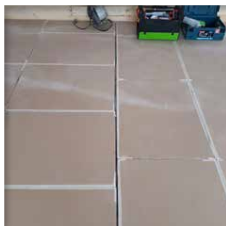
PhoneStar 25 - as a Floor weight improvement board
