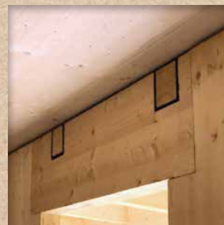
PhoneStrip can also be used as a shadow gap
