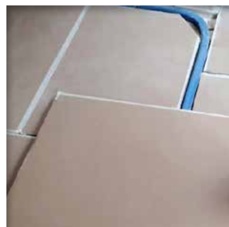
PhoneStar 25 - as line level / height compensation
