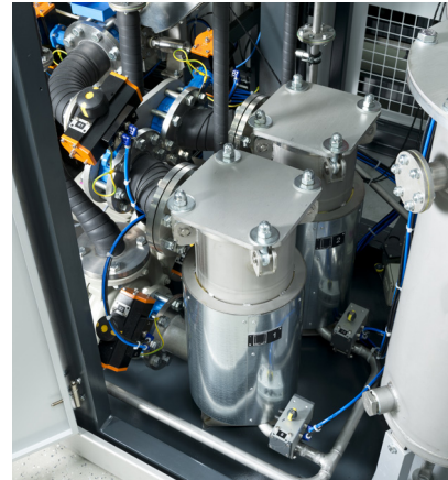
Filter monitoring and drying
