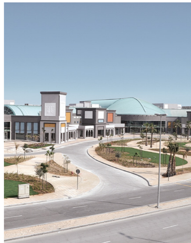
Deira Water Front Market in Dubai The fish market is fully kitted out with 2000 emergency luminaires. The system is protected by a power supply system backed up by battery.
