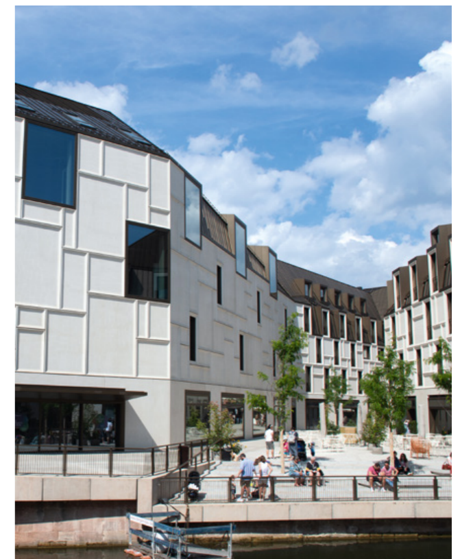
Augustinerhof in Nuremberg Since being opened in 2021, the Augustinerhof is home to the Deutsches Museum as well as hotels, shops and eateries. 950 luminaires and 11 central battery systems from the RP Group are used in the 23 000 m 2 complex.
