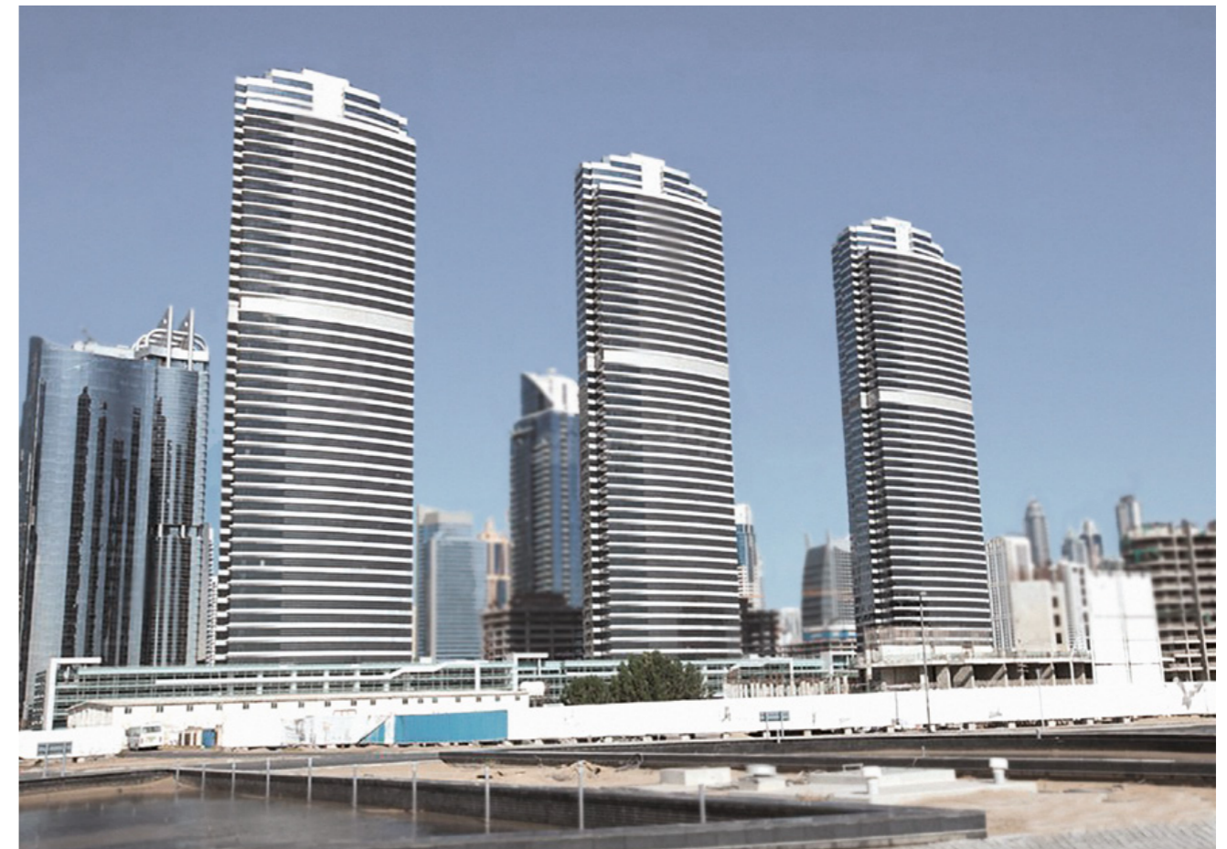
Mazaya Residence in Dubai For superlative safety: completely furnished with 1200 emergency luminaires, protected by a power supply system backed up by battery.
