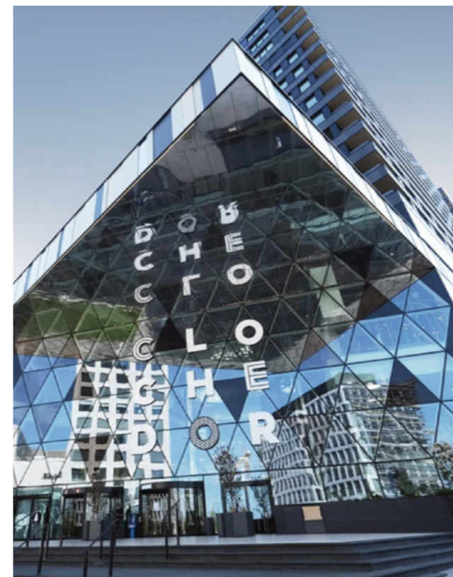
Cloche d'Or in Luxembourg The ultramodern shopping centre (opened in 2019) with 75 000 m 2 of retail space is fitted with around 5000 RP products, including more than 4600 safety luminaires and 9 central battery systems.
